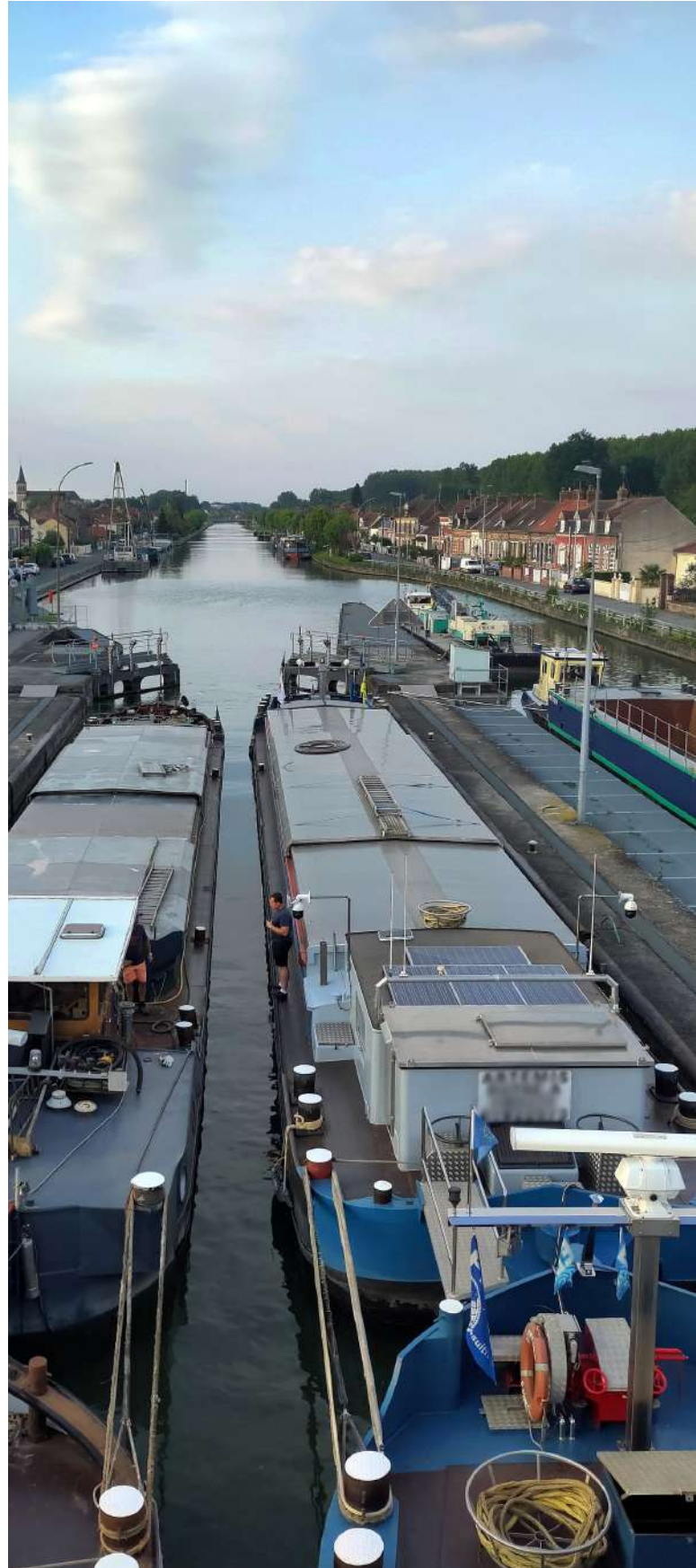
Barges passing through a lock at Compiègne, France.
